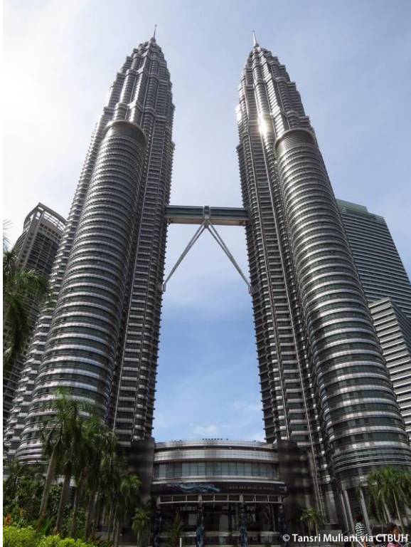
Petronas Towers, Kuala Lumpur (towers appear to be tilted towards each other from a distance)
